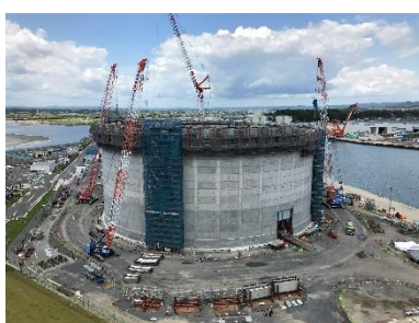
Full View of the Under Construction Tank
